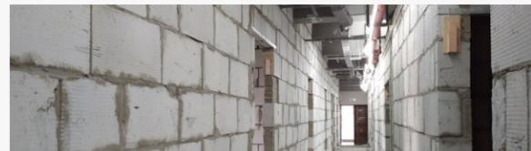
Walls built with eco-friendly aerated concrete bricks
